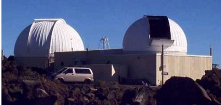
Figure 4.2-7. The HOLLAS Station Mount Haleakala, Hawaii .
