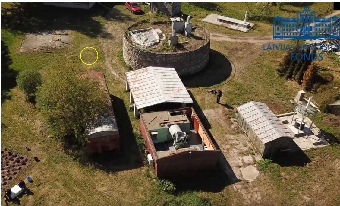
Figure 8-70. Riga station view: The SLR system, GNSS antenna, new local network markers (lower right, top right and near the GNSS antenna) and groundwater monitoring well (yellow circle). Between the SLR and the lower right marker is the old AFU-75 satellite photo camera shed.
