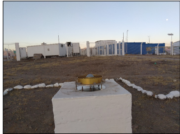
Figure 8-12. GNSS antenna installation at site.
