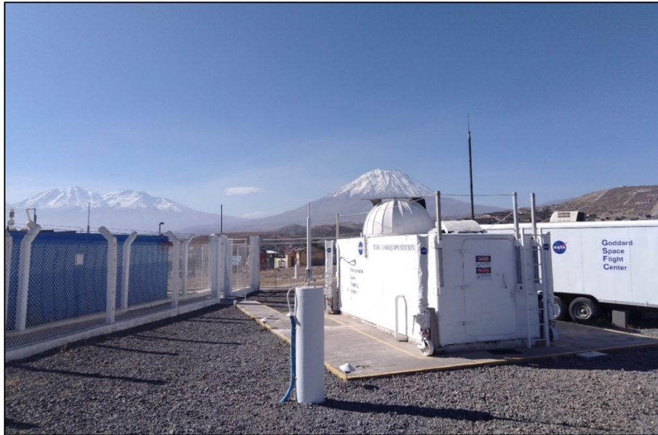
Figure 8-6. TLRS-3 NASA station in Arequipa, with DORIS antenna in foreground and the Chachani and Misti volcanoes in the background.
