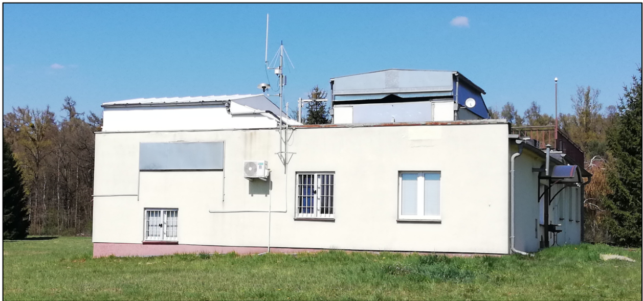
Figure 8-20. The Borowiec system building.
