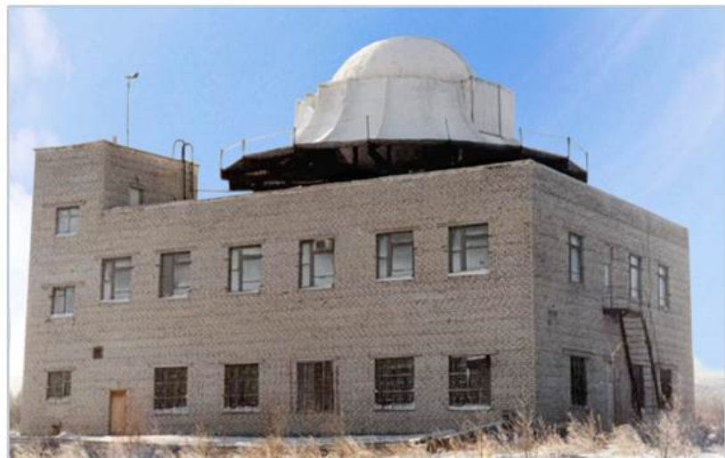
Figure 8-48. SLR system and facility located in Komsomolsk, Russia.
