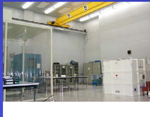
Clean Room for Integration & Test (cleanness : 100,000, 150 sqm)
