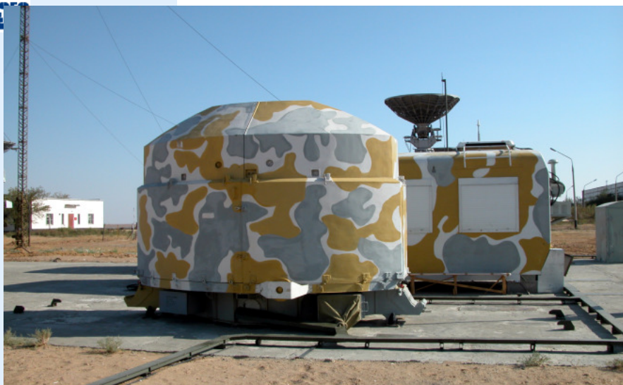
Mobile station under housing
