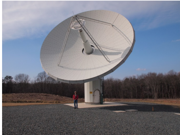
Figure 3: Prototype VGOS antenna at GGAO.
